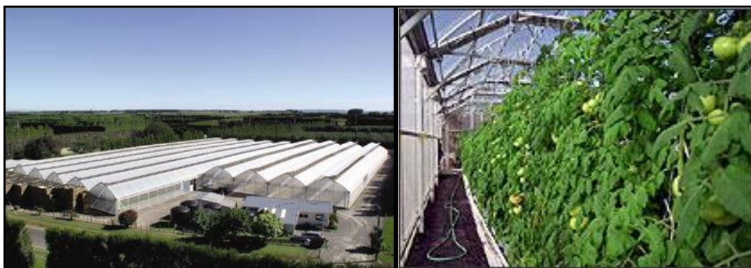
Figure 17: Greenhouses suitable for geothermal heating
